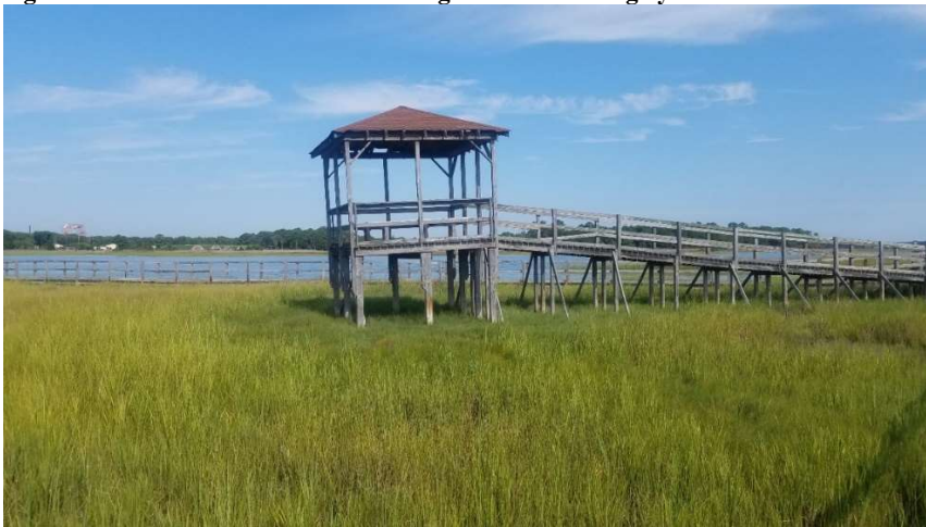
Figure 5: Nature Trail Platform sinking into JBLE-Langley Marsh
